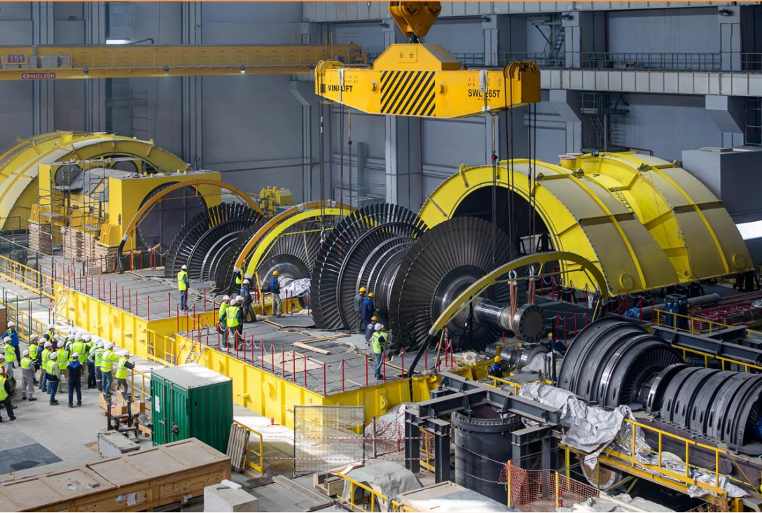
Installation of the Arabelle turbine at the first unit of the Akkuyu nuclear power plant, 2024
